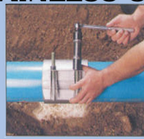
TIGHTEN NUTS EVENLY WITH WRENCH
