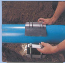
WRAP CLAMP AROUND PIPE
