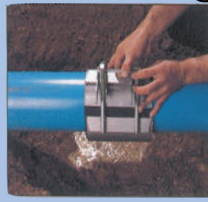
BRING TOGETHER USING LOCKING WASHER PLATE
