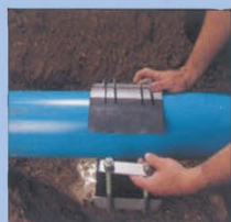
WRAP CLAMP AROUND PIPE
