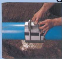
BRING TOGETHER USING LOCKING WASHER PLATE
